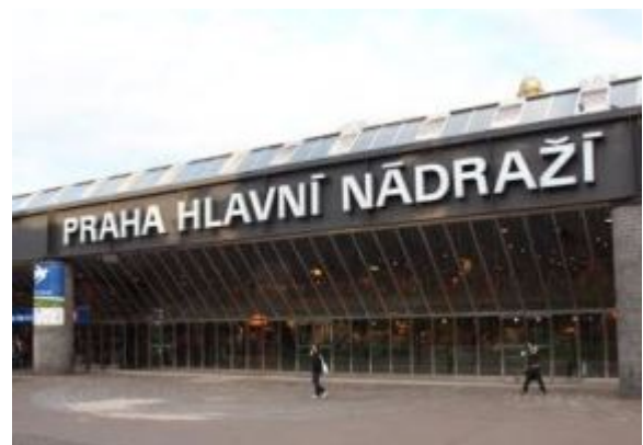
Figure 2.2: Entrance to Main Station
